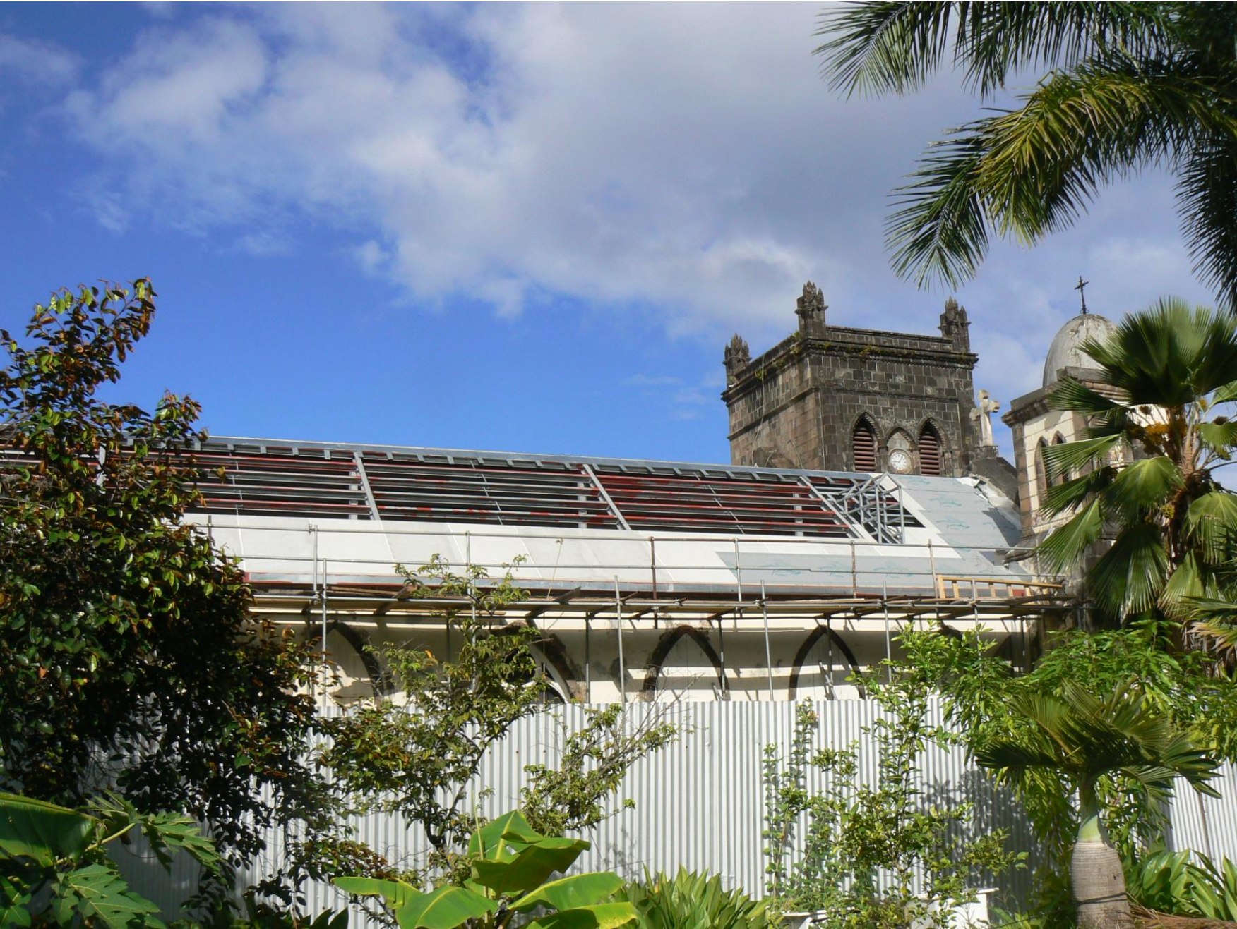
June 2017 : the roofing works continue
