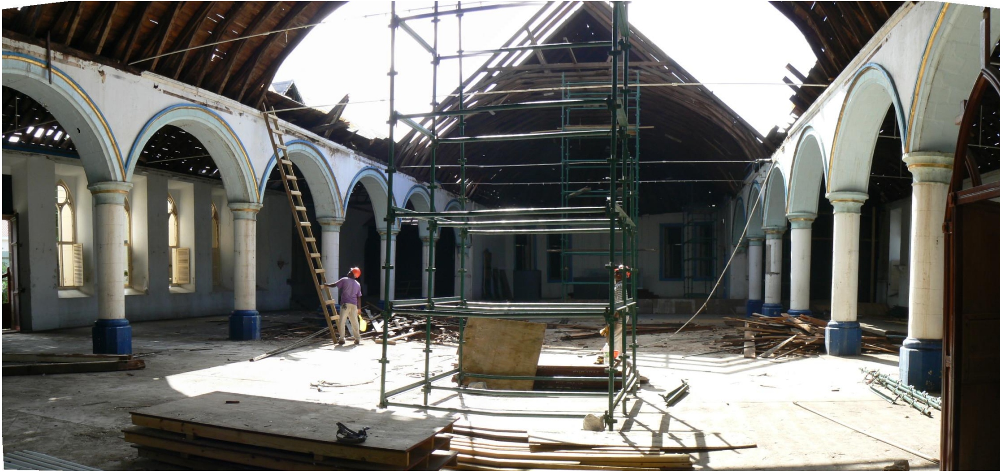
DEMOLITION WORKS FEBRUARY 2013
