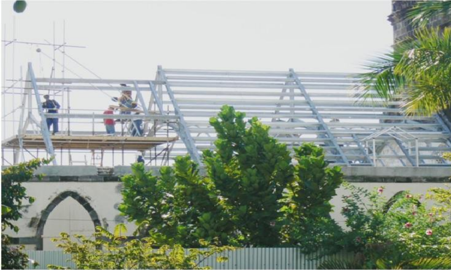
status roof structure December 17, 2014
