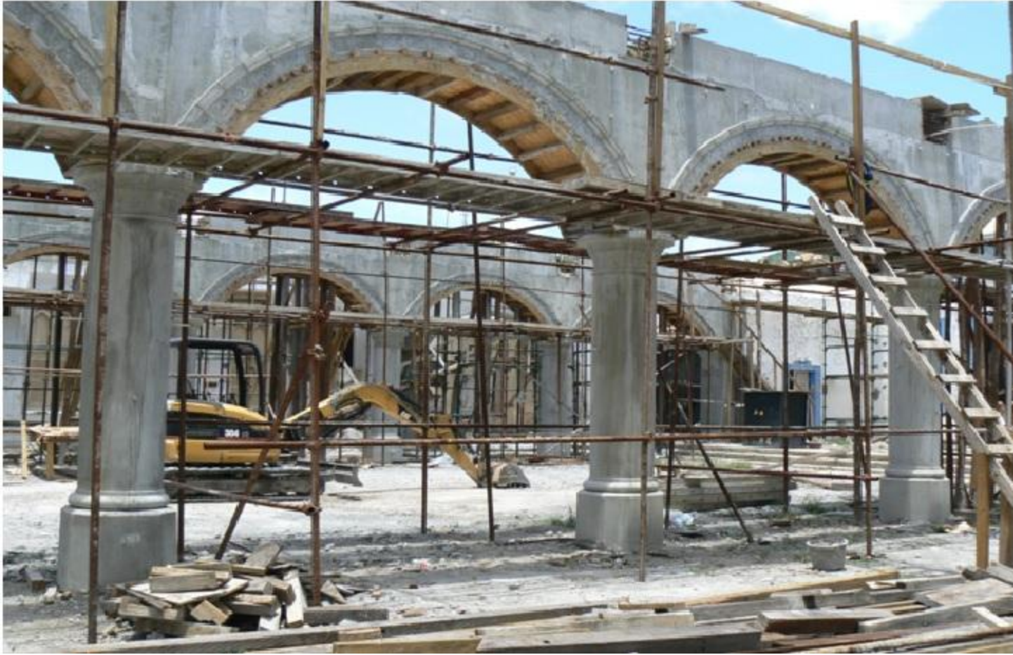
Arches and pillars completed MAY 2014
