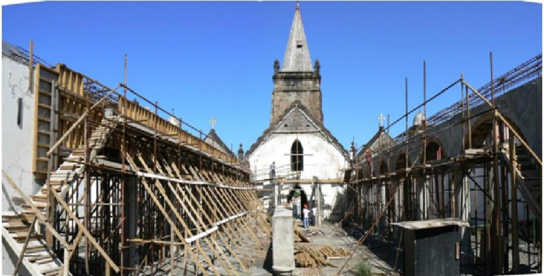
ARCHES and PILLARS in progress MARCH 2014
