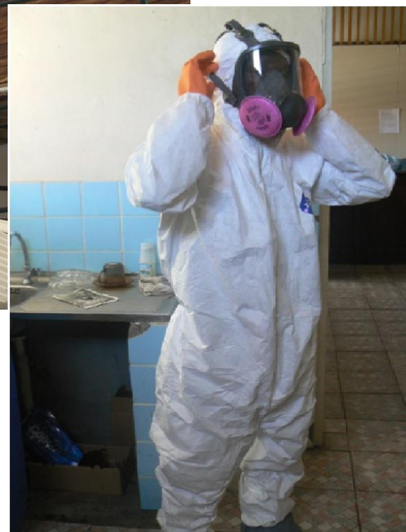
July – September 2012 : removal of roof tiles containing asbestos fibres
