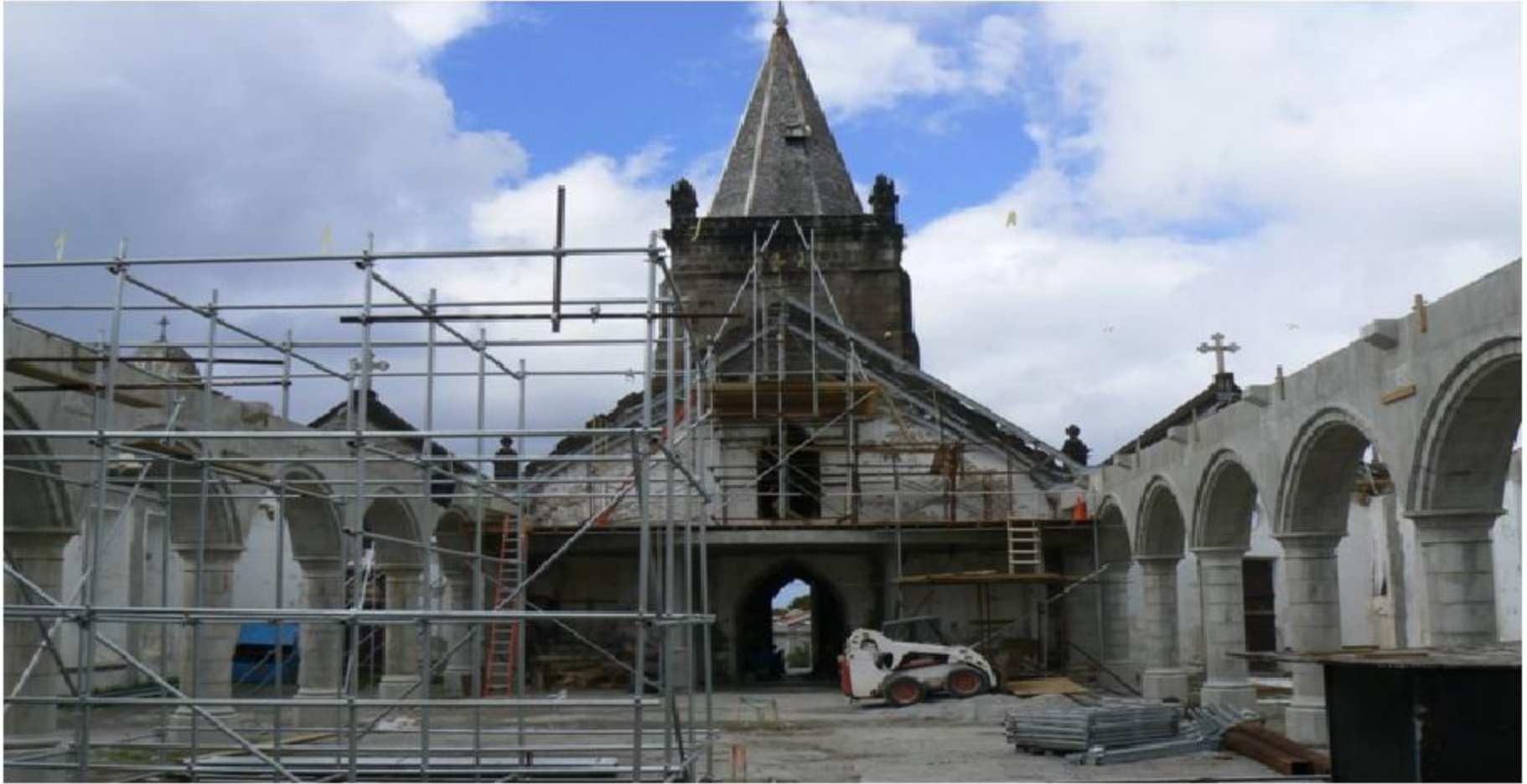
Start on the steel framed roof structure November 2014
